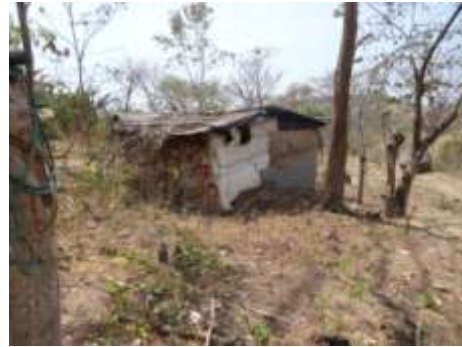
The irrigation project will improve the economic well being of poor farm families on remote settlements.
